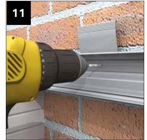
Drill through the wallplate main body and directly through each carriage to suit the masonry anchors being used (not supplied). Mark the position of each masonry anchor on the house wall and drill the house wall to suit.
