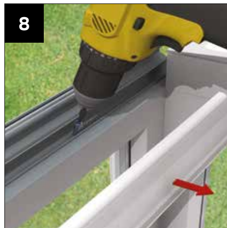
Drill a 5mm pilot hole in the head of the frame, fasten down using 4.8 x 32mm screws (not supplied) at 450mm centres. Refit internal claddings. If fastening up through the frames into the eaves beam use 4.8 x 55mm screws.
