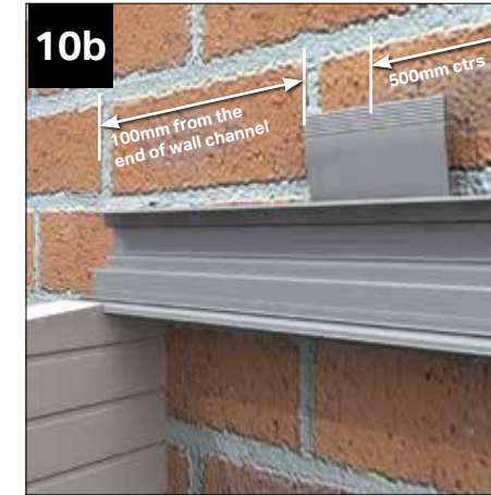
Offer the wallplate up to the wall and position it so that the top surface of the bolt slot is level with the top of the firrings.
